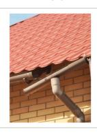
Gutters are have broken in some places. Replace section or repair it. No major damage to it though. 2
