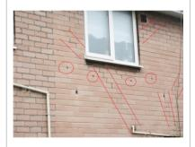
External wall has a cavities and cracks, and repairing it is recommended.
