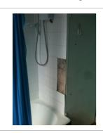
Damaged tiles. Several tiles have broken off of the wall. Could create a sharp surface - hazard. Replace tiles. 3
